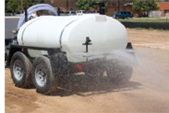
Tow-behind water buffalo providing water mist for dust suppression
